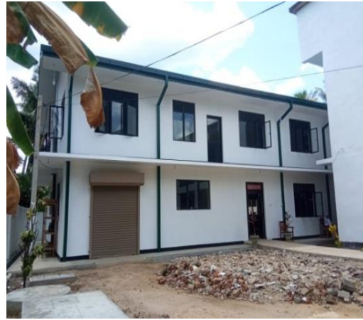
District/Magistrate Court Building, Akkareipaththu
