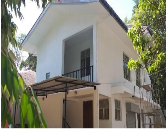
Magistrate Court Building, Rambodagalla
